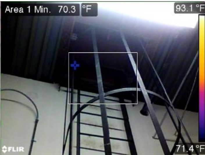
Ladder to roof
