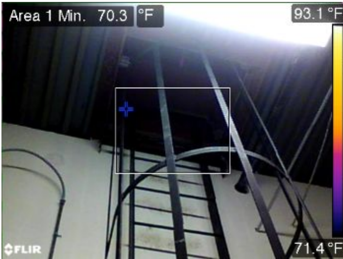
Ladder to roof
