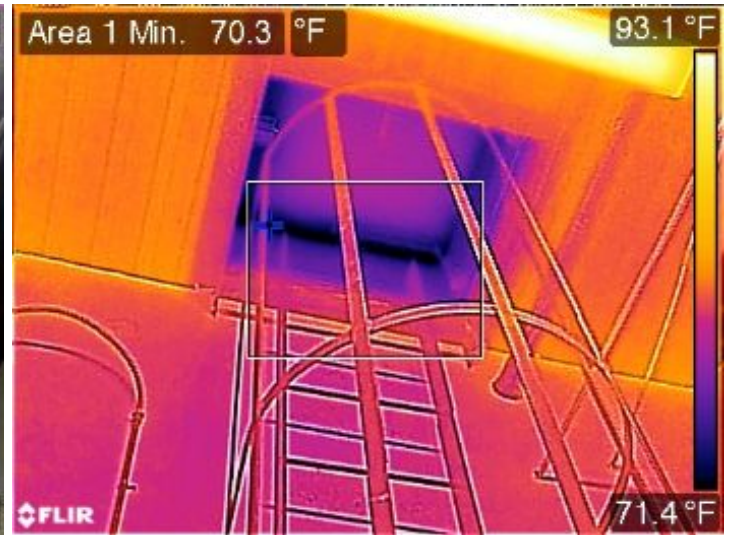
Ladder to roof
