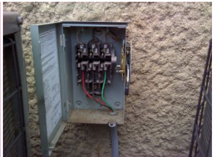
Condenssor disconnect
